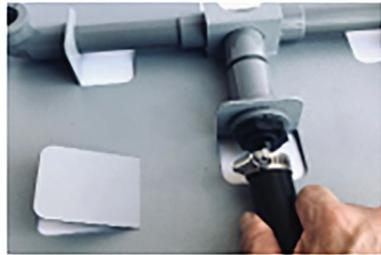
3. Slide hose clamp back over tubing and fasten with screwdriver or nut driver.
